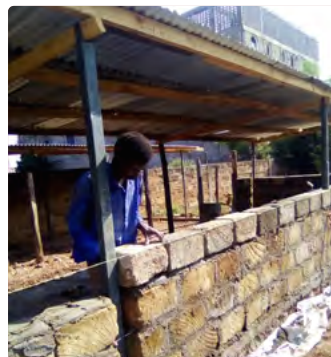
Construction of the cow shed
