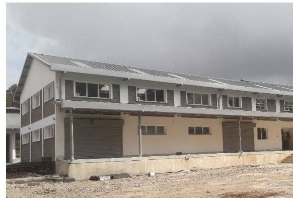
The dairy processing facility, nearly completed
