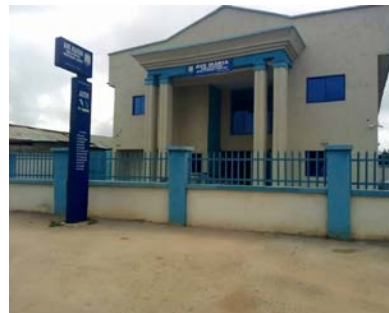
(Above) AMMIL Headquarters
