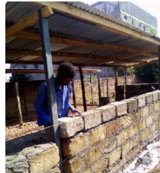
Construction of the cow shed
