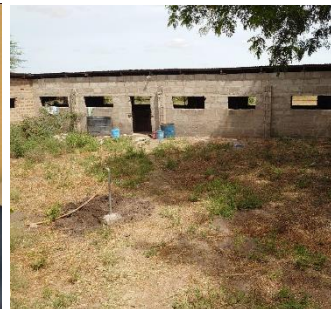
A view from outside the existing pigsty
