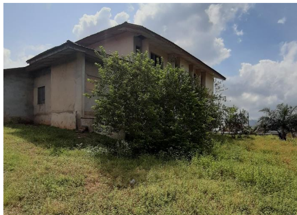
(Above) Kings and EPIS Hostel under construction
