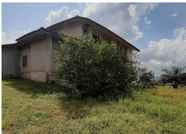
Kings and EPIS Hostel under construction
