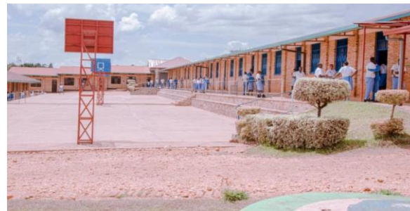
Basketball courts on the school grounds
